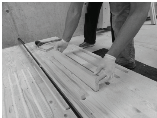
Figure 4. Gluing process: KERTO-S cleats are being inserted into conical slots.
